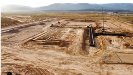
Pictured above, the new GOEX building is being anchored by a utility tunnel that runs under the extrusion area, providing easy access to all mechanical systems and allowing for a clean, unencumbered production floor.
